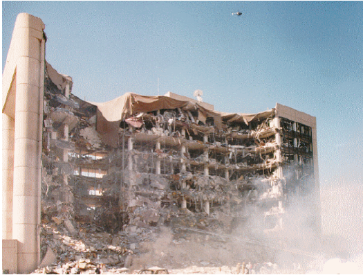
blast induced structural collapse
