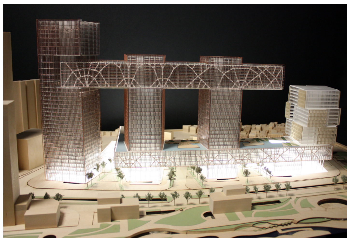
Picture of physical model using topology optimization results (courtesy of SOM) and resemblance to spider webs
